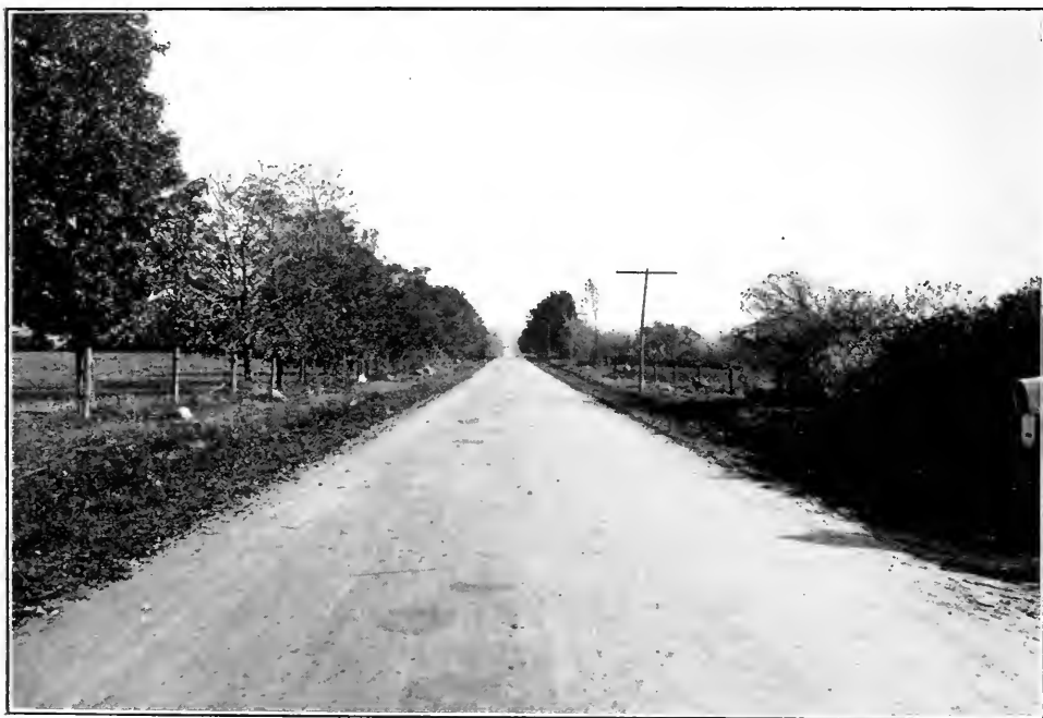
Surface treated macadam road and patched with cold mixture.
